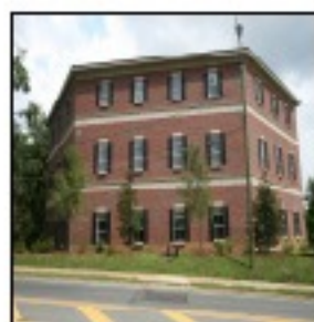
Back of Building
